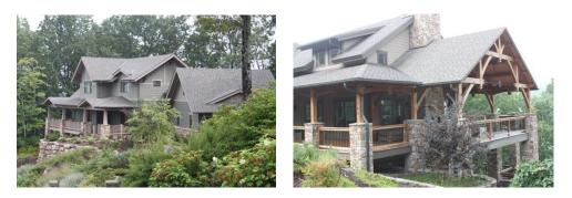
Exposed porch ceiling materials shall be tongue and groove, bead-board, board and batten, and/or exposed rafters, and constructed of wood, cementitious fiber, other composite materials, or other DRB-approved material. Porch ceilings must be either stained or painted with a DRB-approved color.
