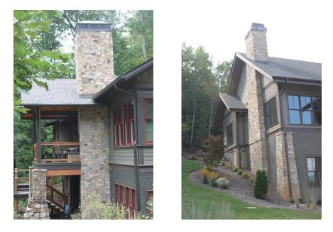
Metal fireboxes are permitted when encased by a masonry veneer. If a fireplace insert is used, the spark arrestor shall be painted flat black and surrounded by a stone, metal chimney cap or other cover approved by DRB. Exposed galvanized caps are not allowed.
