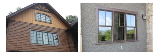
Exterior materials used for window frames, muntins and mullions shall be wood, aluminum, fiberglass, or other cladding as may be approved by the DRB. A muntin (glazing bar) is a small bar that separates two pieces of glass and divides the window into multiple lites. A mullion is a bar or post that separates two window or door units.
